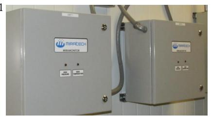
The system is composed of: a monitor, a DP transducer, a temperature transmitter and a Type-K thermocouple. The system operates on 120 VAC. The DP transducer and the temperature transmitter send 4-20 mA signals to the monitor for recording. The system has high temperature and high DP alarms. Data is stored in the monitor for easy download via a Compact Flash Card, USB cable or Ethernet connection to the facilities existing data network. The system can also be configured for MODBUS communication.
