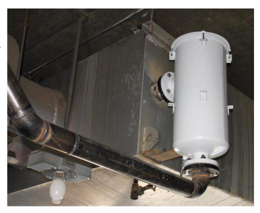
The semi-positive displacement blower pulls a vacuum on the engine crankcase to collect the oil mist and emissions gases for entry into the reclassifier. Inside the reclassifier, the oil mist is separated from the gases and particulates. The oil mist condenses in the bottom of the assembly and is returned to the engine for reuse which reduces engine oil consumption. The filtered, oil free, crankcase gases are then discharged through the plant wall.
